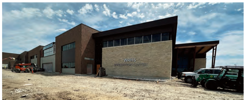
The Innovation Center at Washburn Rural High School
